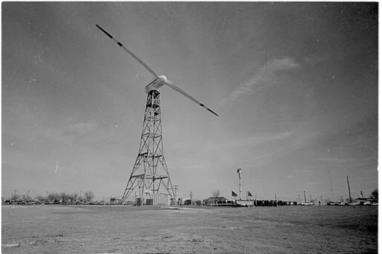
Clayton New Mexico wind turbine dedication, January 1978
